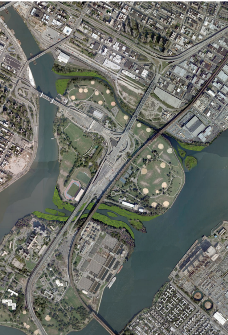
Restoration of Little Hell's Gate
